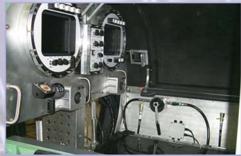
Dolphin Class Integrated Bridge System
